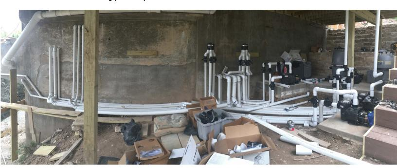
The first few knife edge pools I built, we used a 3" vertical pipe spaced roughly every 5" within the overflow channel. Each of these vertical drop-ins had a 1.5" vent line that that tee d off and returned to the channel. This vent line may be the single most important part of the plumbing because it allows the air to escape the pipe on not create a vacuum. If the draining water creates a vacuum, you will have an immense amount of noise and gurgling escaping the pipe!
