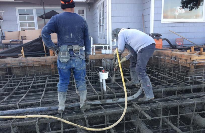
being shot. If you have a hard time convincing your crews to do this, then using a vibrator should help to consolidate the mix. set up soaker hoses on a timer and start keeping the shotcrete moist. Always follow the minimum 2 weeks of curing time before turning off the soaker hoses.
