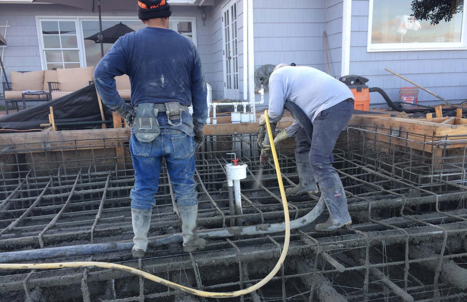
being shot. If you have a hard time convincing your crews to do this, then using a vibrator should help to consolidate the mix. set up soaker hoses on a timer and start keeping the shotcrete moist. Always follow the minimum 2 weeks of curing time before turning off the soaker hoses.
