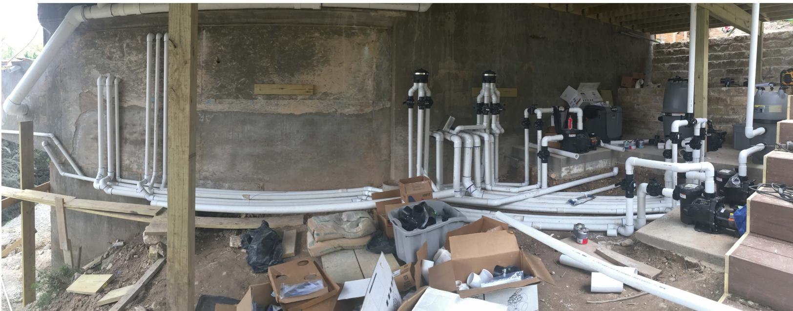
The first few knife edge pools I built, we used a 3" vertical pipe spaced roughly every 5" within the overflow channel. Each of these vertical drop-ins had a 1.5" vent line that tee'd off and returned to the channel. This vent line may be the single most important part of the plumbing because it allows the air to escape the pipe or not create a vacuum. If the draining water creates a vacuum, you will have an immense amount of noise and gurgling escaping the pipe!
